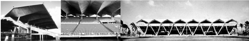
FIG. – 1: Perspective, partial front and back elevation of the Miami Marine Stadium (Miami, Florida 1962 designed by Hilario Candela and Jack Meyer) (Photo courtesy Friends of the Miami Marine Stadium http://www.marinestadium.org/ ).
