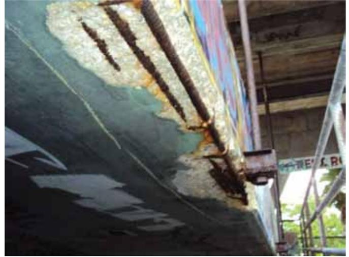
**Fig. 5:** Deterioration in mezzanine slab at hanger location (photo courtesy of SGH)
