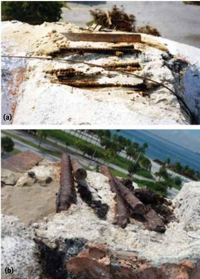
**Fig. 8: Deterioration of post-tensioning anchorage zone of the diaphragm end: (a) 1993; and (b) 2009** (photos courtesy of SGH)
