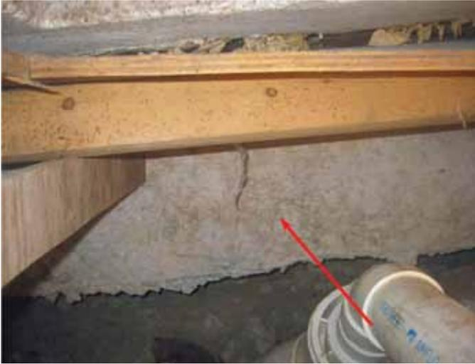
**Fig. 4:** The undersides of the slabs and grade beams are in good condition (photo courtesy of SGH)
