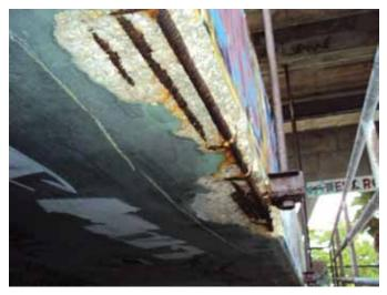
Fig. 5: Deterioration in mezzanine slab at hanger location (photo courtesy of SGH)
