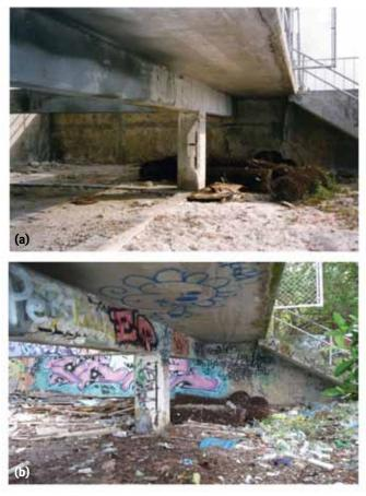
Fig. 9: Column showing increased spalling: (a) 1993; and (b) 2009 (photos courtesy of SGH)
