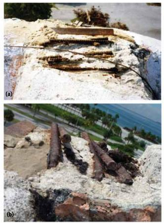
Fig. 8: Deterioration of post-tensioning anchorage zone of the diaphragm end: (a) 1993; and (b) 2009 (photos courtesy of SGH)
