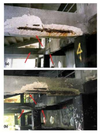
Fig: 10: Beams over water showing growth of spalls and new spalls: (a) 1993; and (b) 2009 (photos courtesy of SGH)
