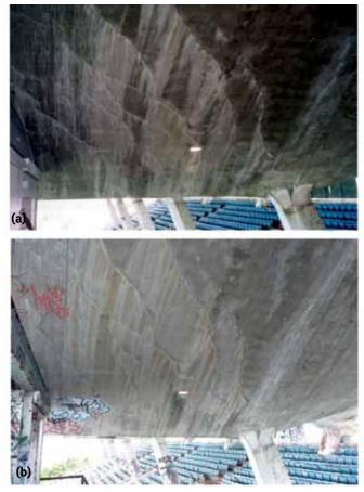
Fig. 7: Cracking on bottom side of roof: (a) 1993; and (b) 2009 (photos courtesy of SGH)
