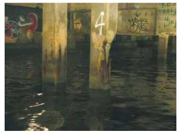
Fig. 3: Concrete piles below the lower seating area show moderate-to-severe deterioration (*photo courtesy of SGH*)
