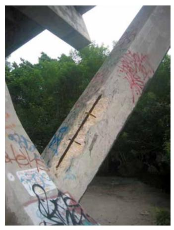
Fig. 6: Deteriorated inclined column (photo courtesy of SGH)
